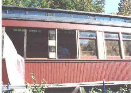
Peeling back the plywood and plastic bit by bit gives a chance to install the outer stops and siding without too much exposure to a
